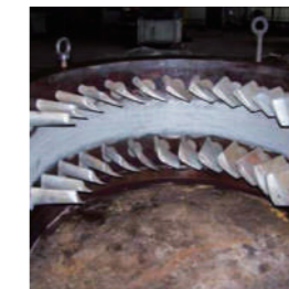
Hydro power guidevane repair
