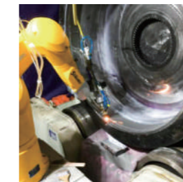
Repair of the inner ring bearing surface of the crane drum
